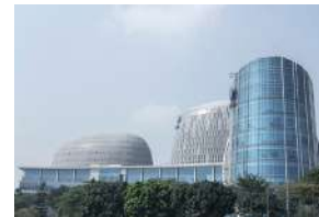
Three Main UMN Building Tiga Gedung Utama Kampus UMN
